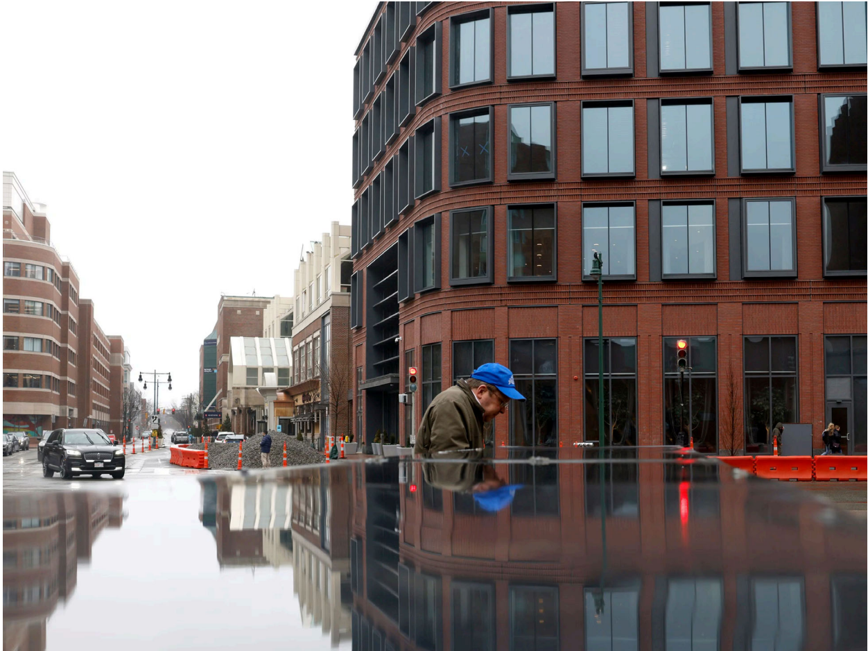
A new lab building was built at the site of the former Macy's at the CambridgeSide Galleria. (JESSICA RINALDI/GLOBE STAFF)
