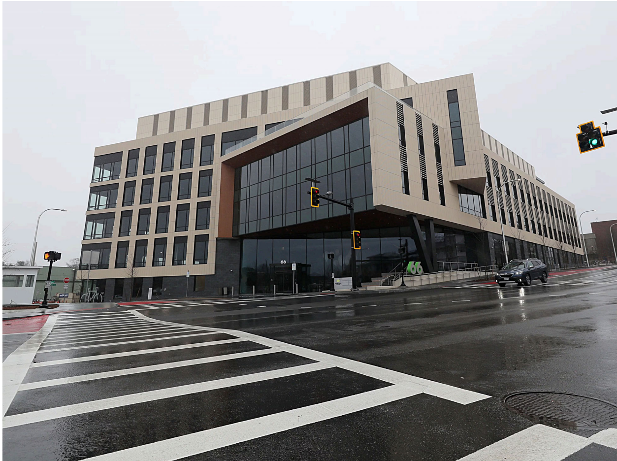
Construction is nearly complete at 66 Galen Street in Watertown. (SUZANNE KREITER/GLOBE STAFF)
