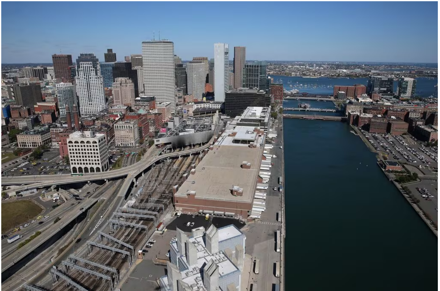
The US Postal Service sorting facility alongside South Station. DAVID L. RYAN/GLOBE STAFF
