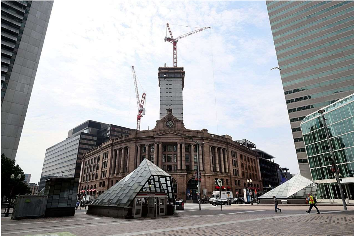
Construction on the tower above South Station. SUZANNE KREITER/GLOBE STAFF
